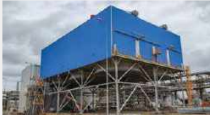
AZERKIMYA—Installation and commissioning of steam turbine
