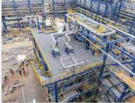
Upgrade and Reconstruction of SOCAR's Heydar Aliyev Oil Refinery (PACKAGE A)
